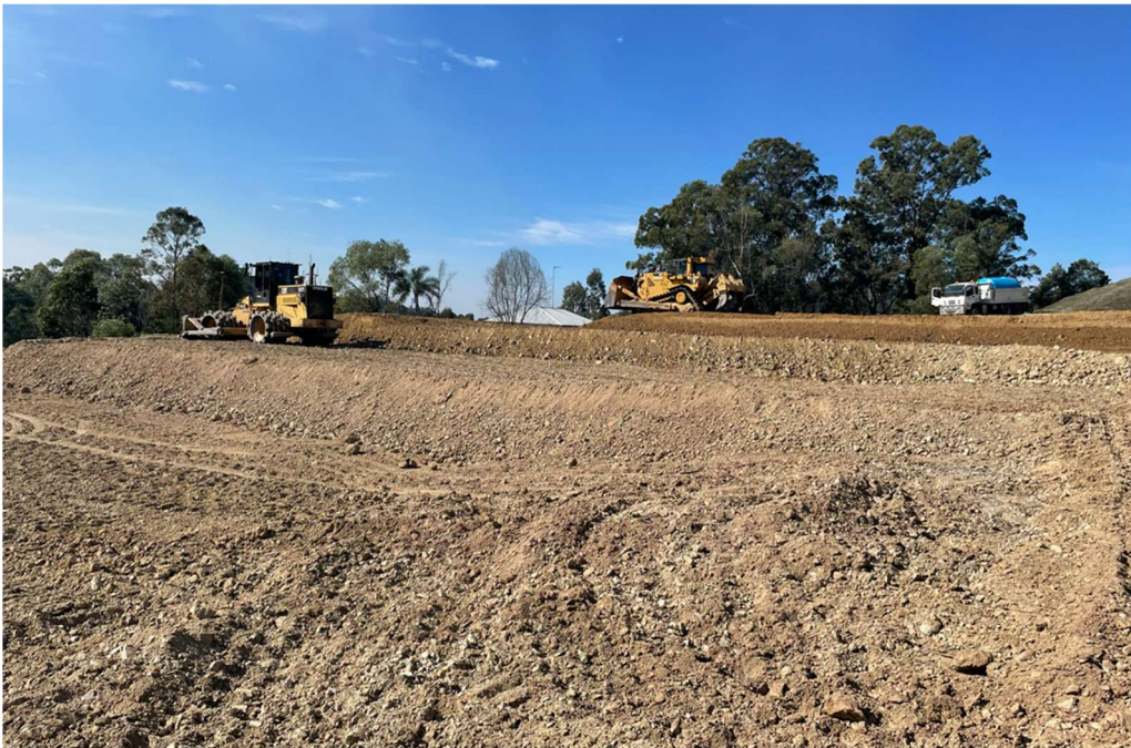
Image D – Compaction of fill material
