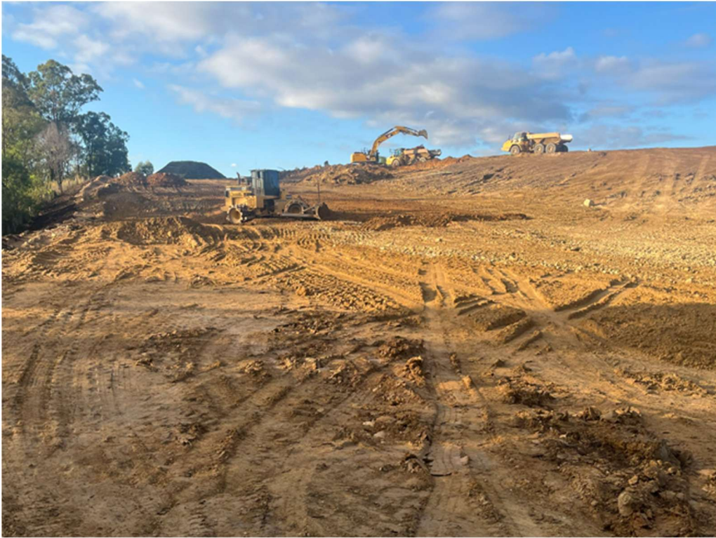
Image C – Compaction of fill material
