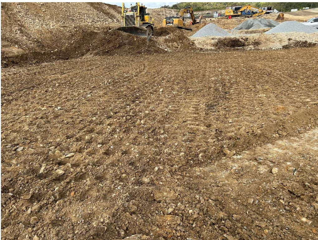
Image F – Compaction of fill material near the finished level
