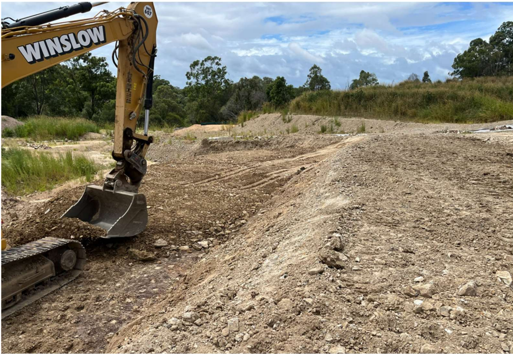
Image E – Trimming of placed fill material
