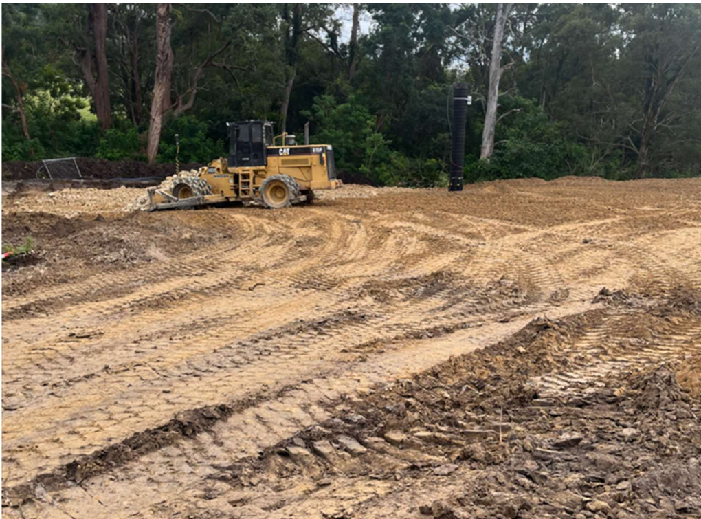
Image B – Compaction of fill material
