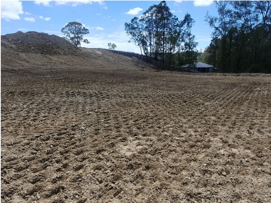
Progress photograph (southern portion of Stage 1) – 11 th December 2023.
