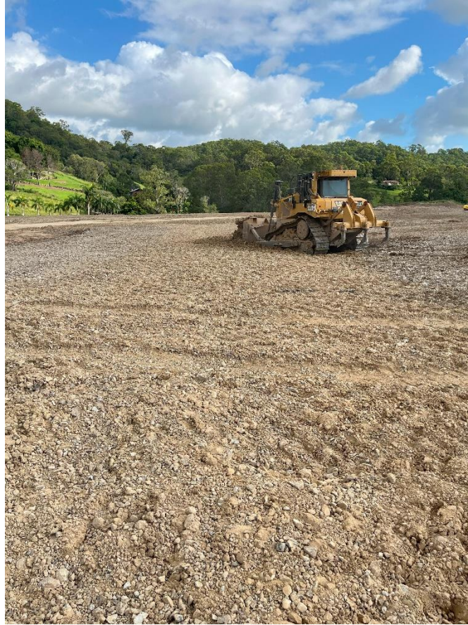
The Stage 1 fill area near the finished surface level.
