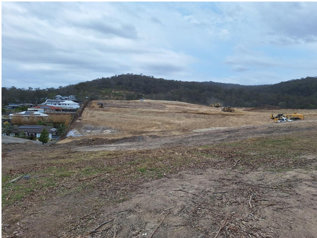
Progress photograph – 1 st November 2023.
