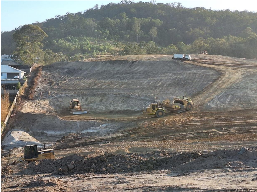
Progress photograph – 25 th October 2023
