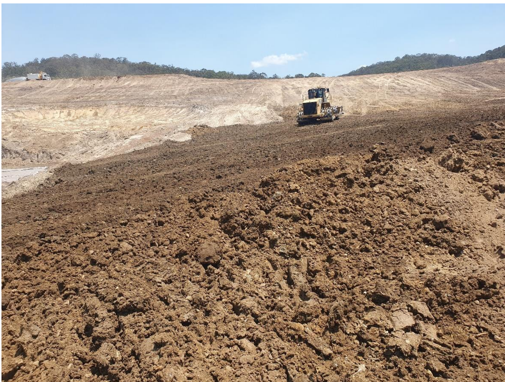
Compaction of the lower fill layers using the Cat 815 compactor.
